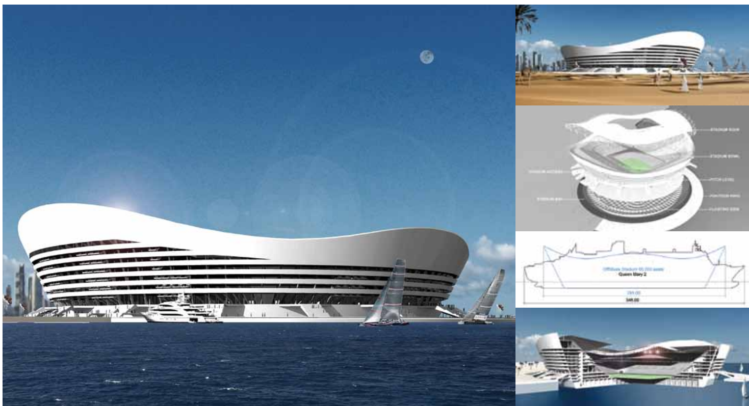
German firms Stadiumconcept and ArenaCom have conceived a 65,000-seater floating off-shore stadium. Approaching the size of the giant cruise liner RMS Queen Mary 2, the stadium would be founded on a large floating disk and constructed using renewable materials. It would include 180 executive boxes
